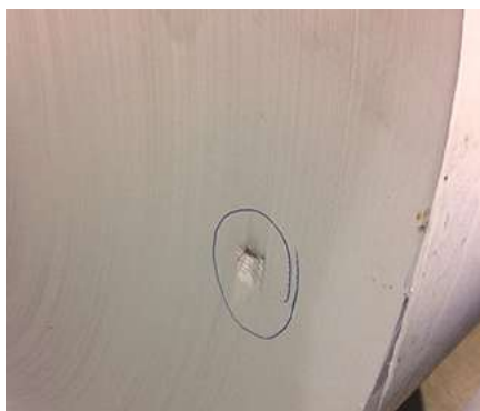
End damage due to debris. Source: Stora Enso.
