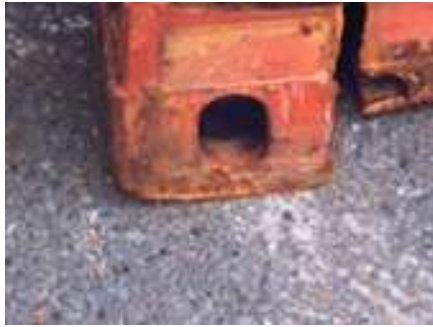
22 Broken front sill.
