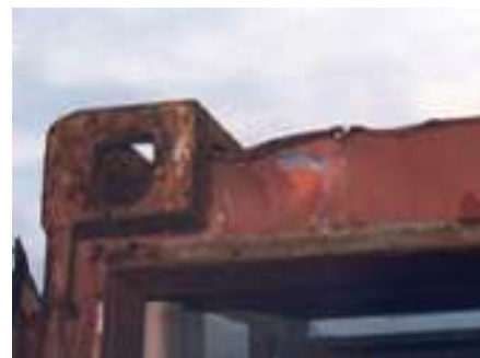
2 Damaged door header.
