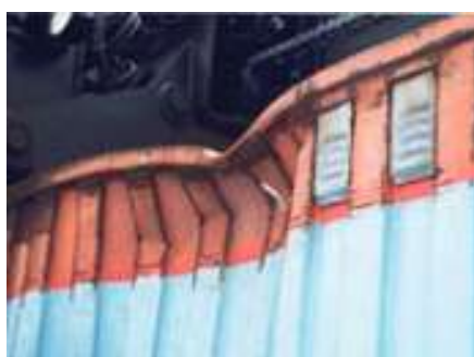
17 Bent top side rail.
