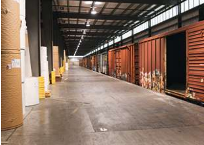
The loading areas for wagons at European paper mills are normally protected against adverse weather conditions. Source: INTAKT.
