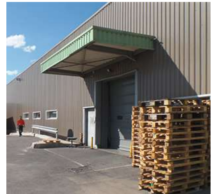
✗ Ground-level loading doors with weather protection showing poor operating practices: Unused pallets should not be stored close to the building where they create a fire risk; the walkway along the outside of the wall is blocked. Source: icmPrint.
