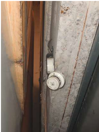
✘ Fire detection systems must be in good condition and not obstructed. Source: IF P&C.
