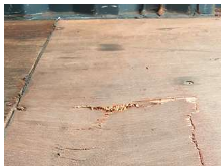
15 Holed plywood floor. Source: Mëtsa Board.
