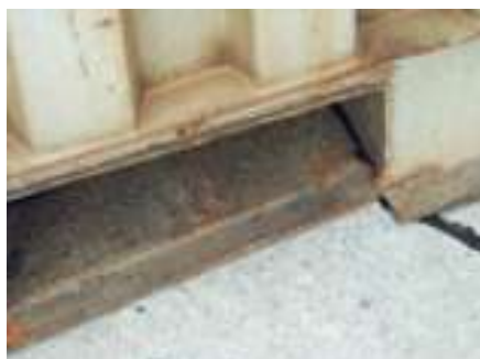
19 Cracked forklift pockets.
