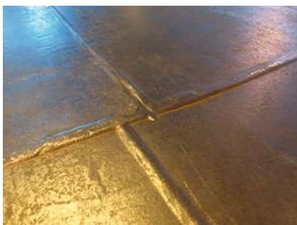
Welded floor seam in hold. Source: UPM.
