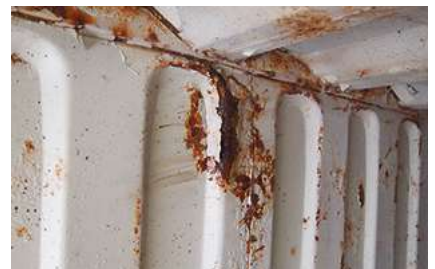
Examples of unacceptable walls. Source: UPM (3.3.8)
