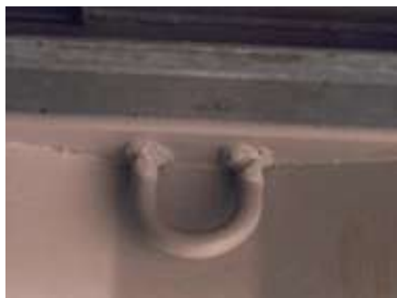
16 Broken lashing fitting.
