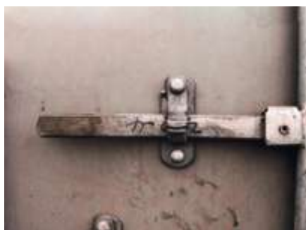
7 Complete door handle retainer and missing handle catch.
