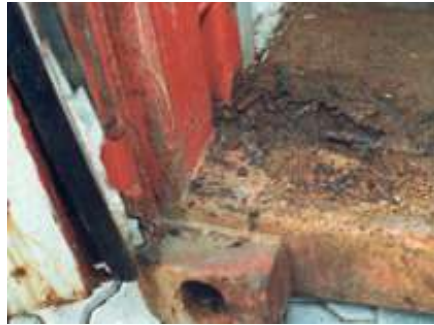
11 Rusted threshold door plate.
