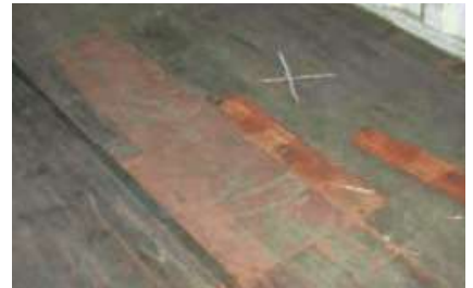
Is the repaired floor strong enough? Source: UPM 3.3.6
