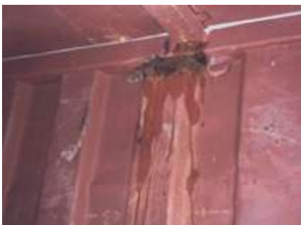
14 Rusted internal roof.
