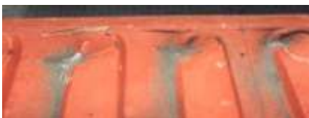
25 Dented external roof.
