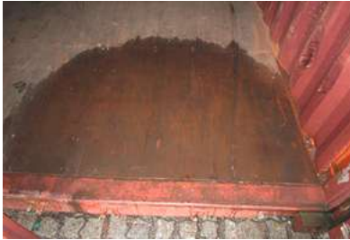
Soiled container floor. Source: Mëtsa Board.
