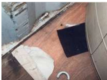
16 Missing bottom lashing fittings.
