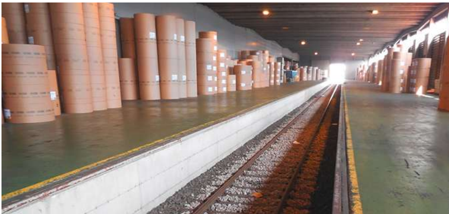
Covered rail platform ensures dry conditions for loading and unloading. Source: IF P&C.
